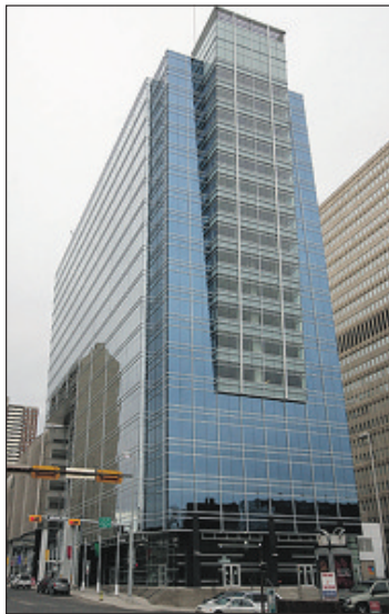
The new Palliser South office tower is ready for occupancy.
